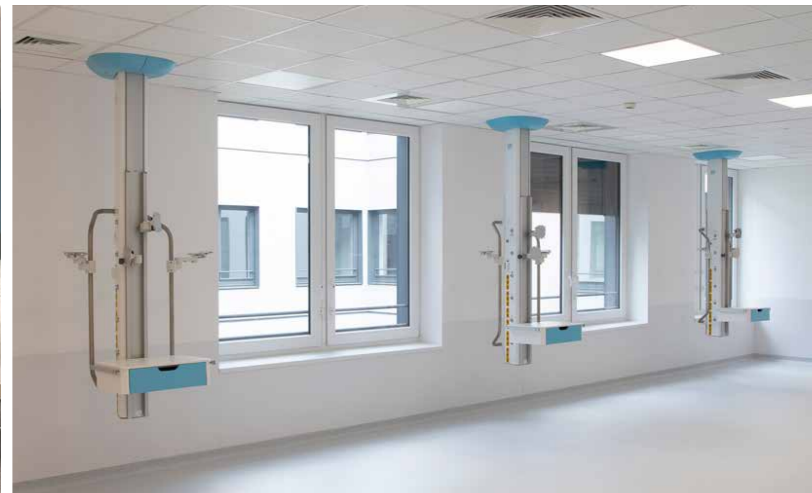
Centre Hospitalier, Maubeuge, France Hospital Center, Maubeuge - France
