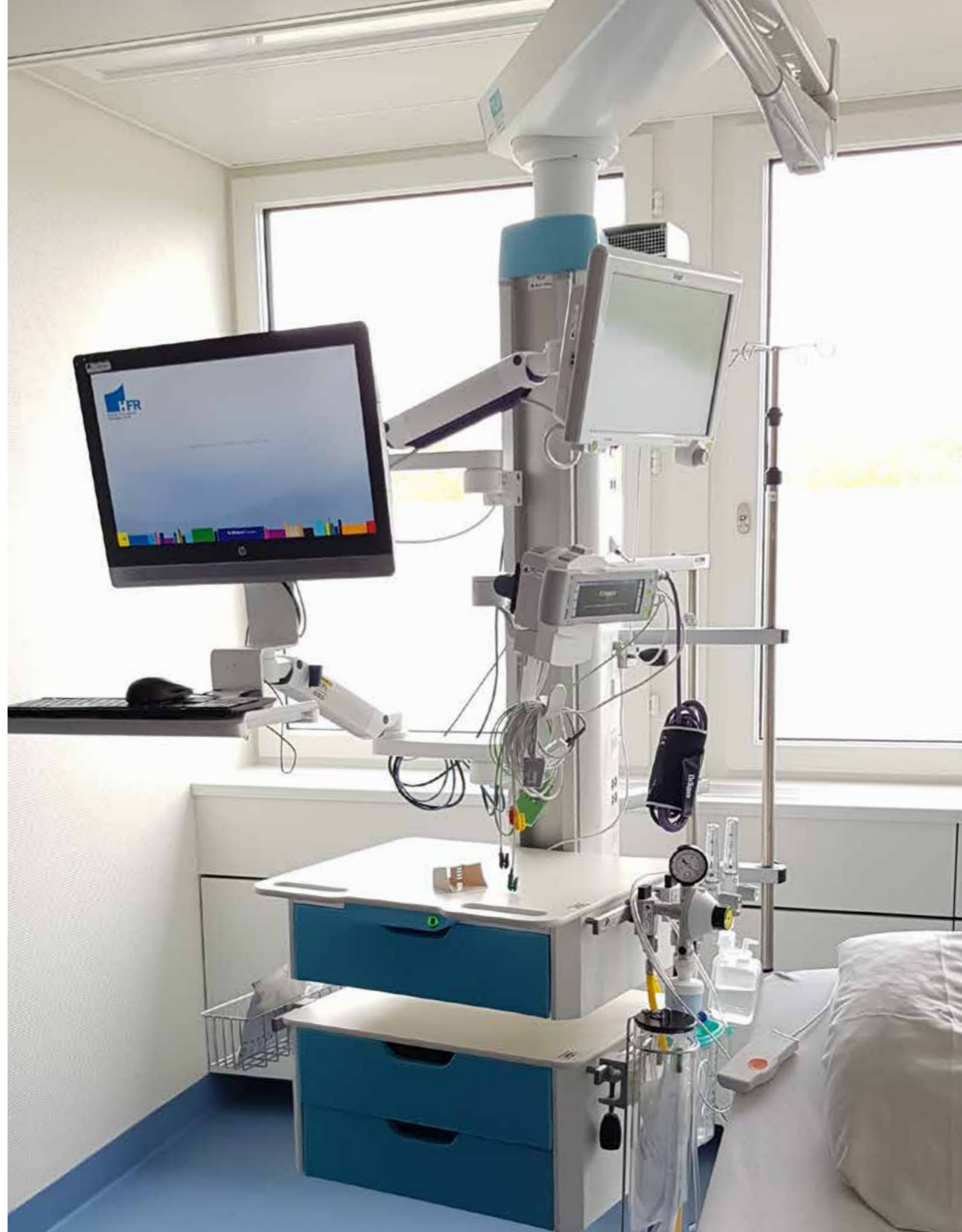
Service des Urgences, Hôpital, Fribourg - Suisse Emergency Department, Hospital, Fribourg - Switzerland
