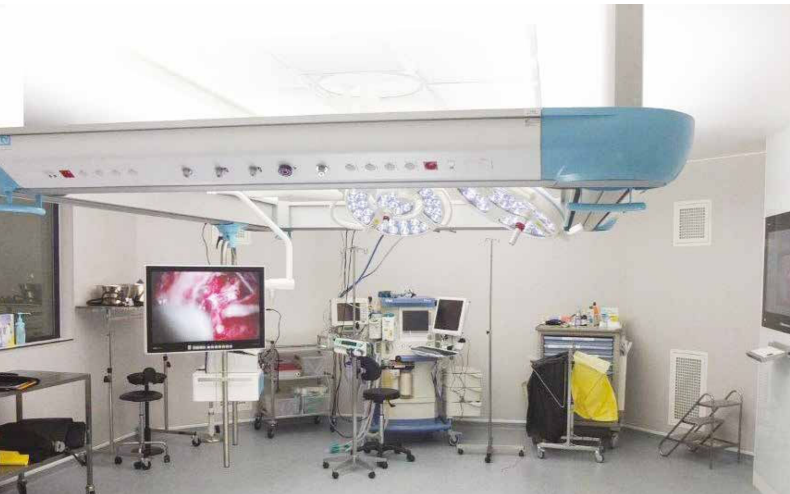
Hôpital Henri Becquerel, Rouen Henri Becquerel Hospital, Rouen - France
