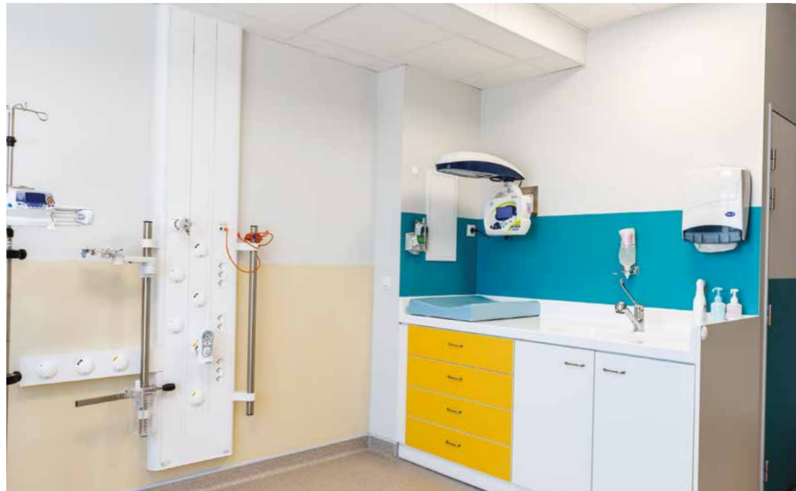
Centre Hospitalier, Annecy Hospital Center, Annecy - France
